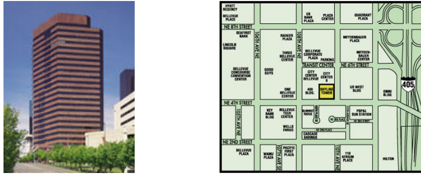
Figure 3. Skyline tower and location
